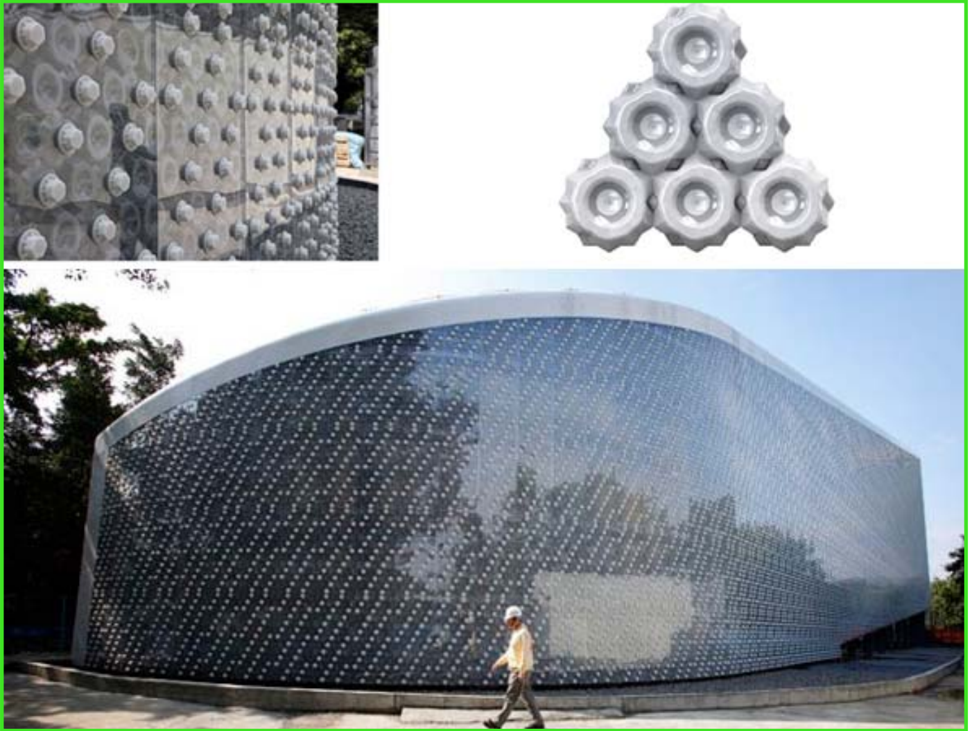
Fig. 5.34: Polli-bricks made from recycled PET bottles can be made to look appealing and modern. (Source: Sundance Channel, 2010)
