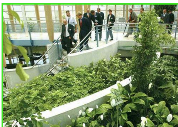
Fig. 5.8: Living Machine installed in an atrium. It looks just like any green feature. (Source: Ecofriend, 2008)
