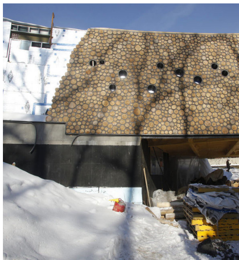
038. Facade going up.
