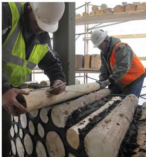
037. Community joins in to build the cordwood facade.
