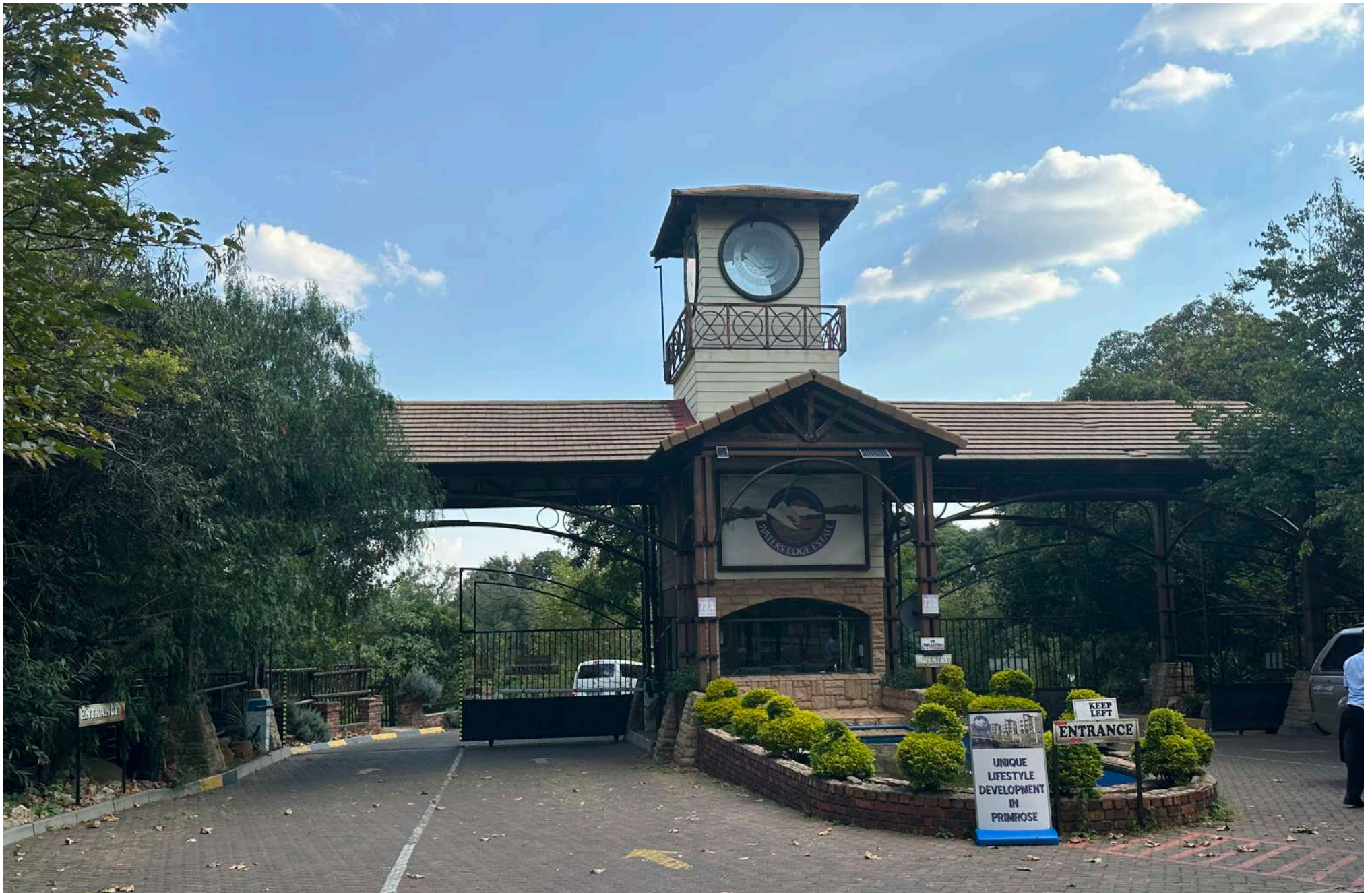
Figure 5.24: Existing Access Control (Author, 2023)
