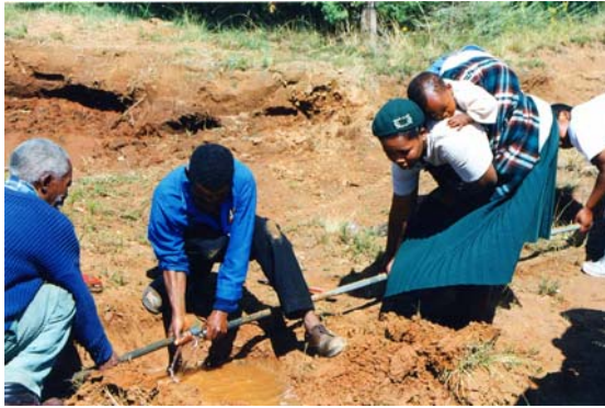
Digging up the pipe to see where possible blockages might be
