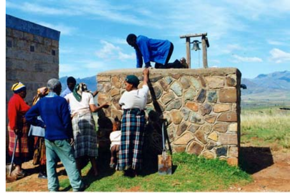
Cleaning out the catchment tank at the primary school
