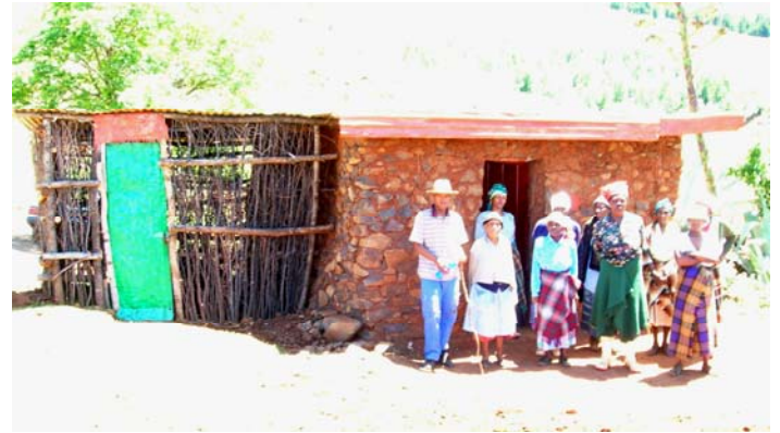
The new stone structure houses the shop while the adjoining shelter is used for circle meetings
