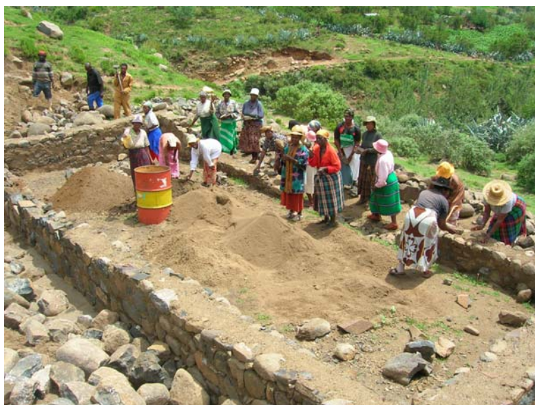
Circle members building a pre-school in Sekhutlong village
