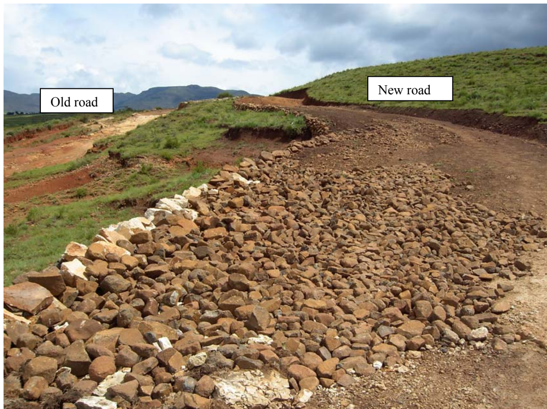
A photo showing the old track alongside the newly constructed road
