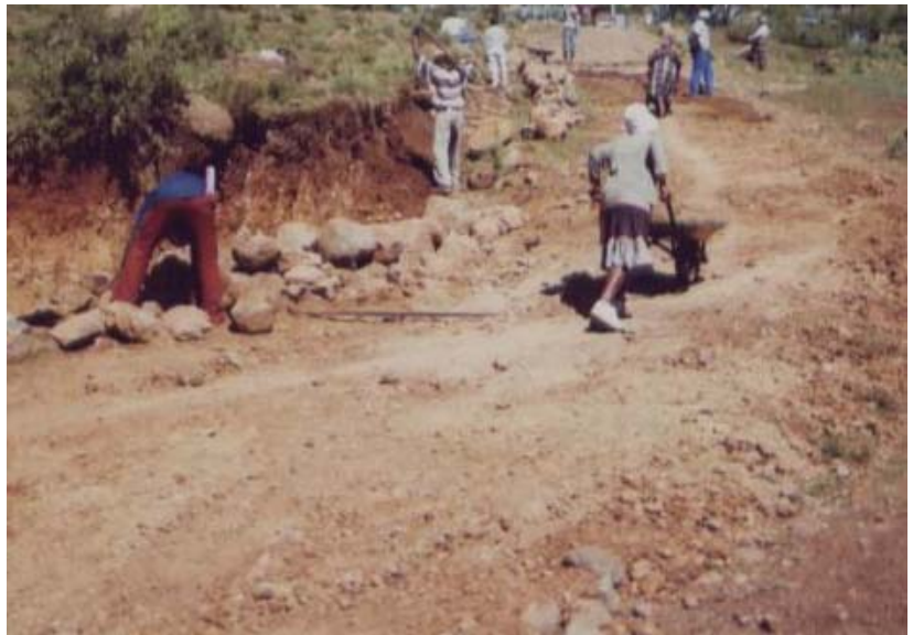
Construction on the road begins
