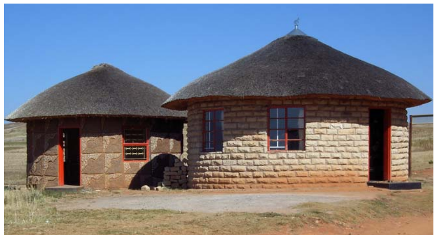
Right front – the new Handicraft Sales Room; Left – the new handicraft work room (Sponsored by the US Embassy in Lesotho)
