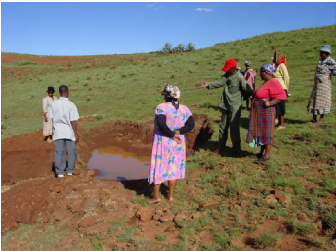
Circle members discussing the excavation of their dam
