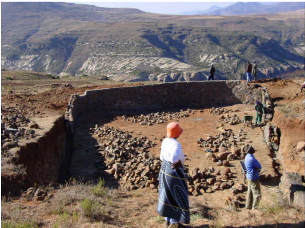
The dam is excavated ... and the walls go up
