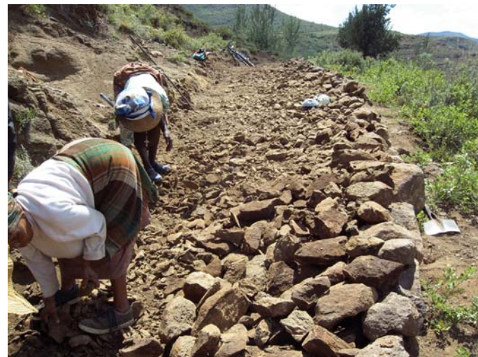
Circle and community members constructing an access road from their village into the valley below
