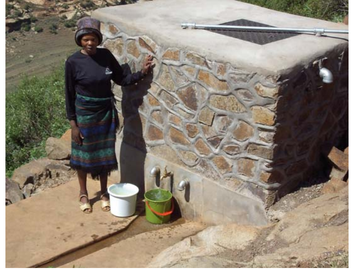
... and after completion of the new protected structure
