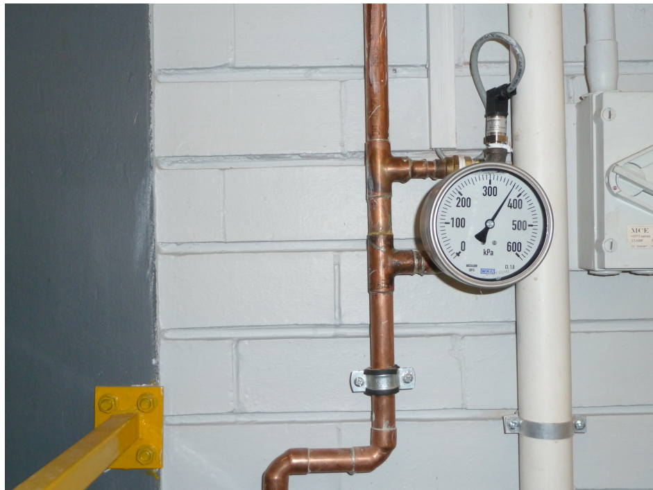
FIGURE A.4: Water inlet pipe with pressure regulator.
