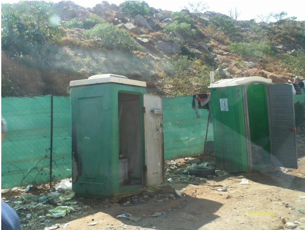
Communal Shared Chemical Toilets
