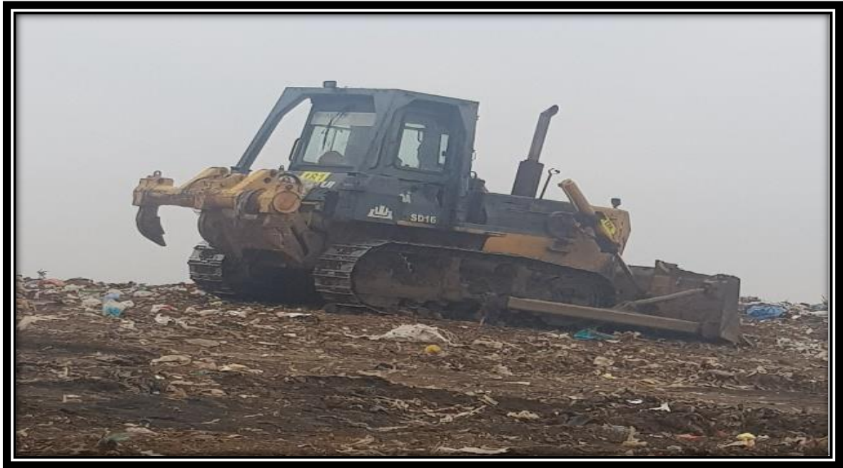
Figure1.5 Equipment used by the contractor (Ngobeni, 2023)
