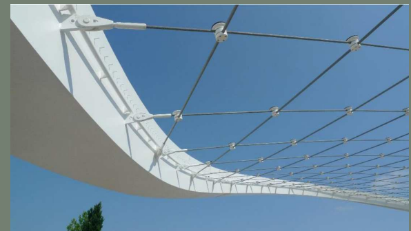
Figure 7.13: Cable and fork connectors with threaded fittings along edge beam.
