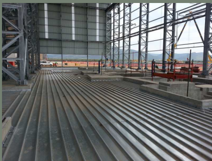
Figure 7.26: Installation of Decking © Global Roofing (2019)
