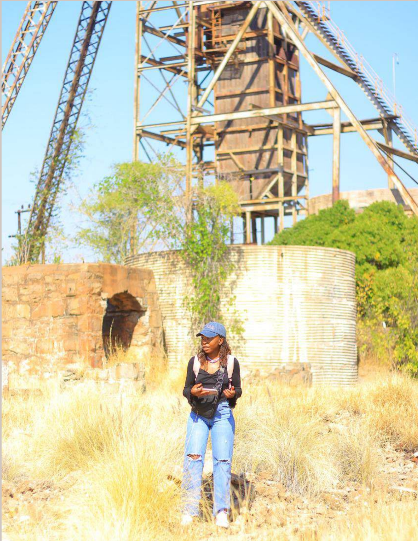
Figure 64: Musina Old Copper Mine shaft Photograph by Chase the photographer (Mr N Mudau) during my site visit in Musina, 13 July 2024.
