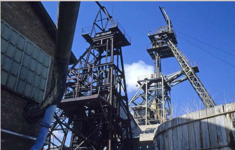
Figure 56: “The two headgear at the Messina Mine. The one in the foreground is the old No 4 shaft that operated from 1906-1918. The taller headgear in the background was the No 5 Shaft” Harper shaft, Messina mining district [WWW Document], n.d. . mindat.org. URL https://www.mindat.org/photo-725598.html (accessed 9.4.24).
