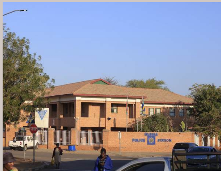
Figure 23: Musina Police Station. Photograph by Chase the photographer (Mr N Mudau) .
