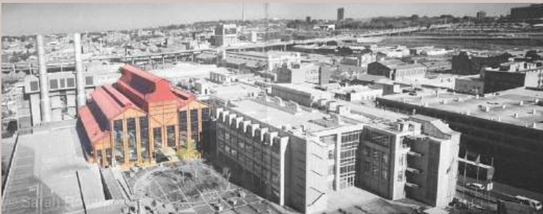
Figure 84: Adaptive Reuse of theTurbine Building and the redevelopment of 1913 Market Hall into a museum. "Seed Crystal" or Cathedral in the Square? Urban Industrial Adaptive Reuse in Contemporary South Africa [WWW Document], n.d. . Society of Architectural Historians. URL https://www.sah.org/publications/sah-blog/blog-detail/sah-blog/2018/10/04/seed-crystal-or-cathedral-in-the-square-urban-industrial-adaptive-reuse-in-contemporary-south-africa (accessed 9.7.24).
