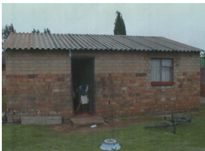
Typical house in Soweto built circa 1960, with an asbestos cement roof.
