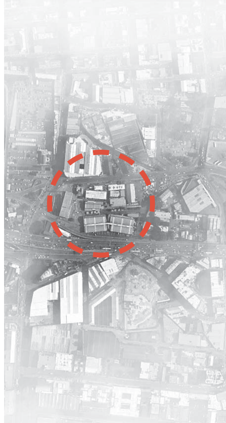
32 Aerial photograph: Faraday Precinct (source: after Google Earth)
