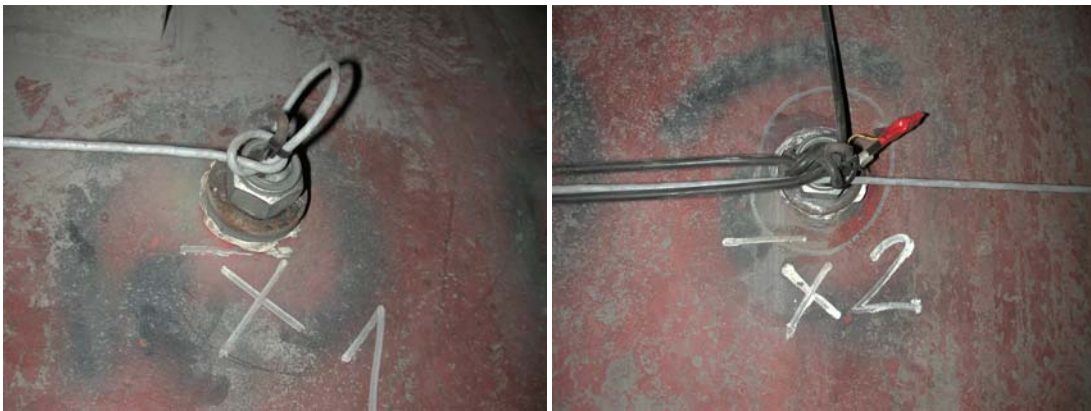
Figure A3.1.2: Conductivity probes CM1 and CM2, installed and connected to control box.
