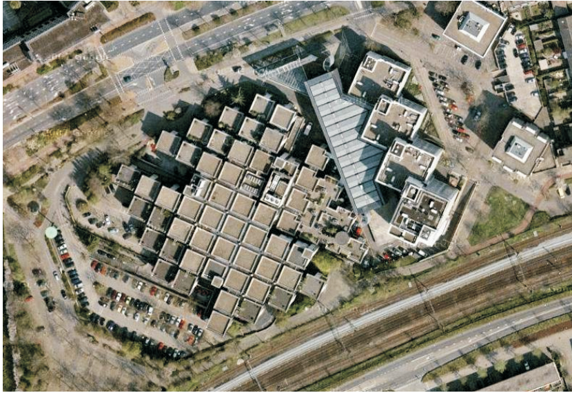
Aerial View of Central Beheer by Hetzberger (www.greatbuildings.com; cited 07/2008)
