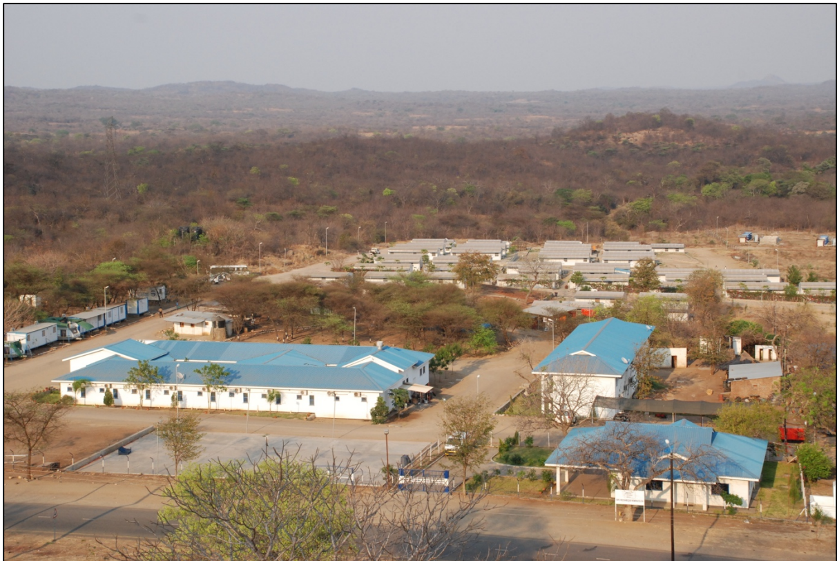
Figure 6 – An overview of the Colony taken from the armed lookout point: the Hospital is in the bottom right-hand corner, with the family homes perpendicularly behind it. The large, blue-roofed rectangular building to the centre left of the image is the guesthouse and dining room. The rows of beige-roofed of barrack-type cabins are where the expats live.
