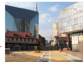
TOP SQUARE ON DIAGONAL STREET
