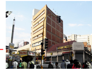
OSKOP HOUSE (BACK) KAZERNE BUILDING (FRONT)
