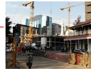
VIEW TOWARDS THE NEW FNB CONSTRUCTION SITE
