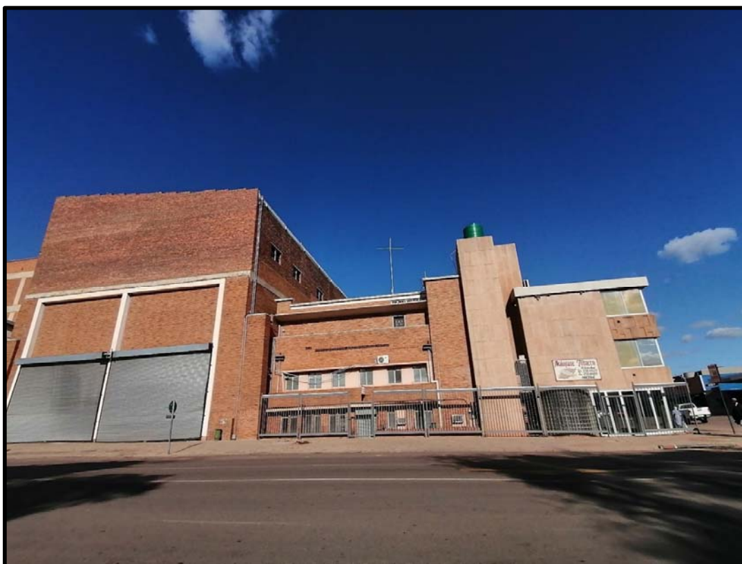
Figure 57: Offices of the old Tobacco Cooperative stand empty today. Photograph taken by author on 4 March 2020.
