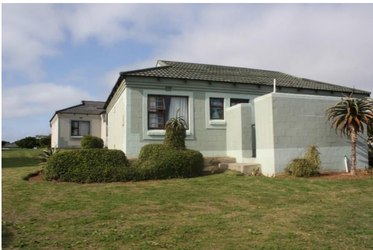
Figure 4.1: taken by the author in 2015 demonstrates a one storey detached house at Vulindlela Accommodation.
