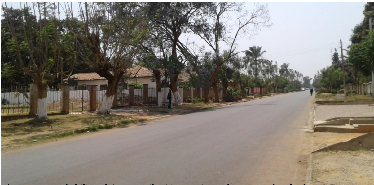
Figure 5.11: Rehabilitated Avenue Likasi in quartier Makomeno Lubumbashi
