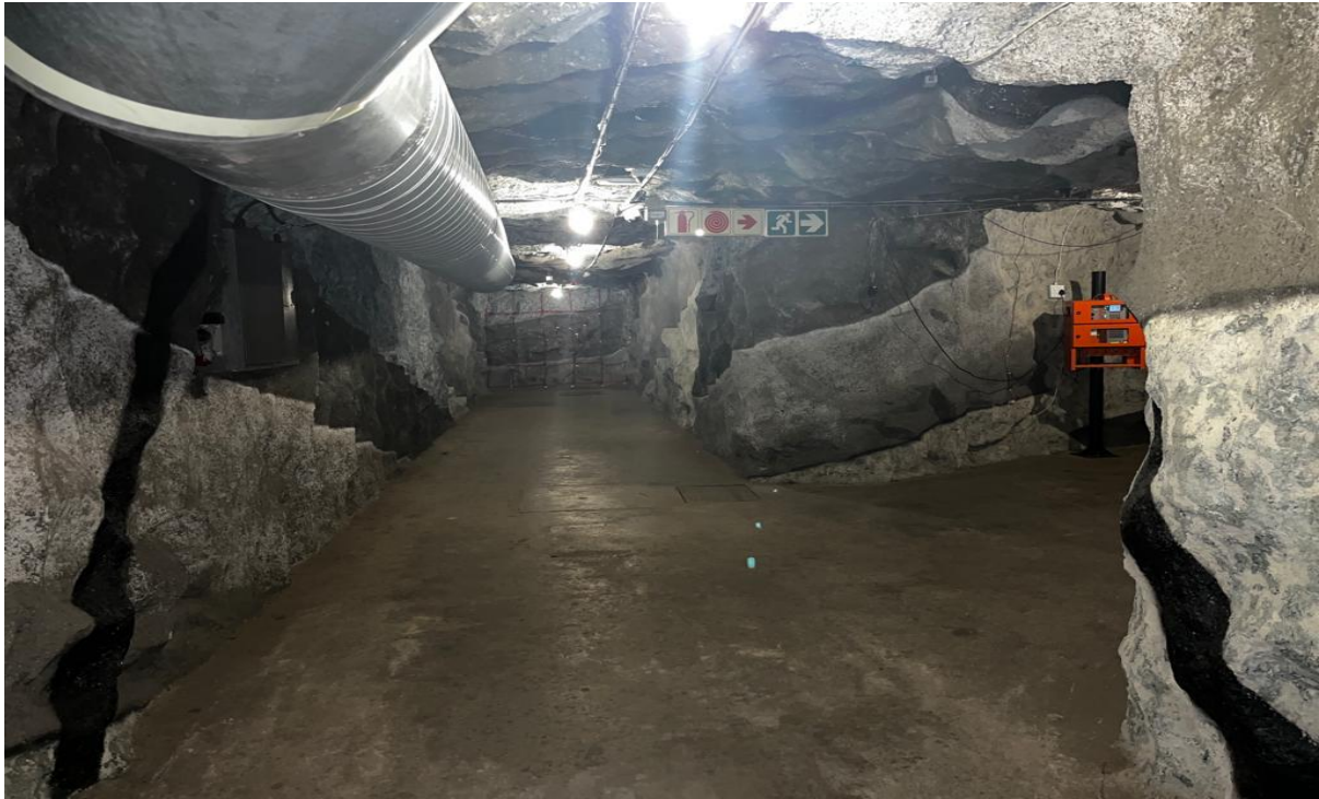
Figure 11: Image of the tunnel displaying rock formations, artificial lighting, ventilation pipe and blasting system.
