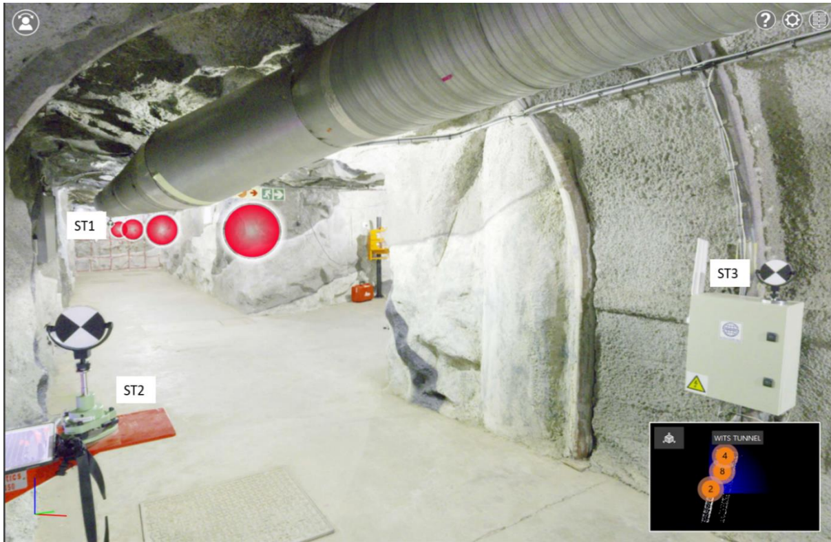
Figure 18: Target network of three tie points (ST1, ST2, ST3) selected for the registration of the laser data
