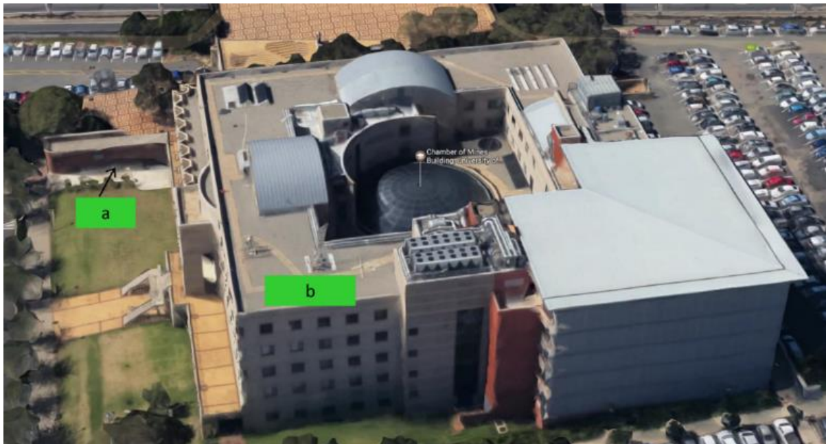
Figure 10: Chamber of Mines building. (a) The mock “underground mine” tunnel at the lower ground section of the building. (b) A weather station situated on the roof of the main building signifies the surface of the mock underground mine.
