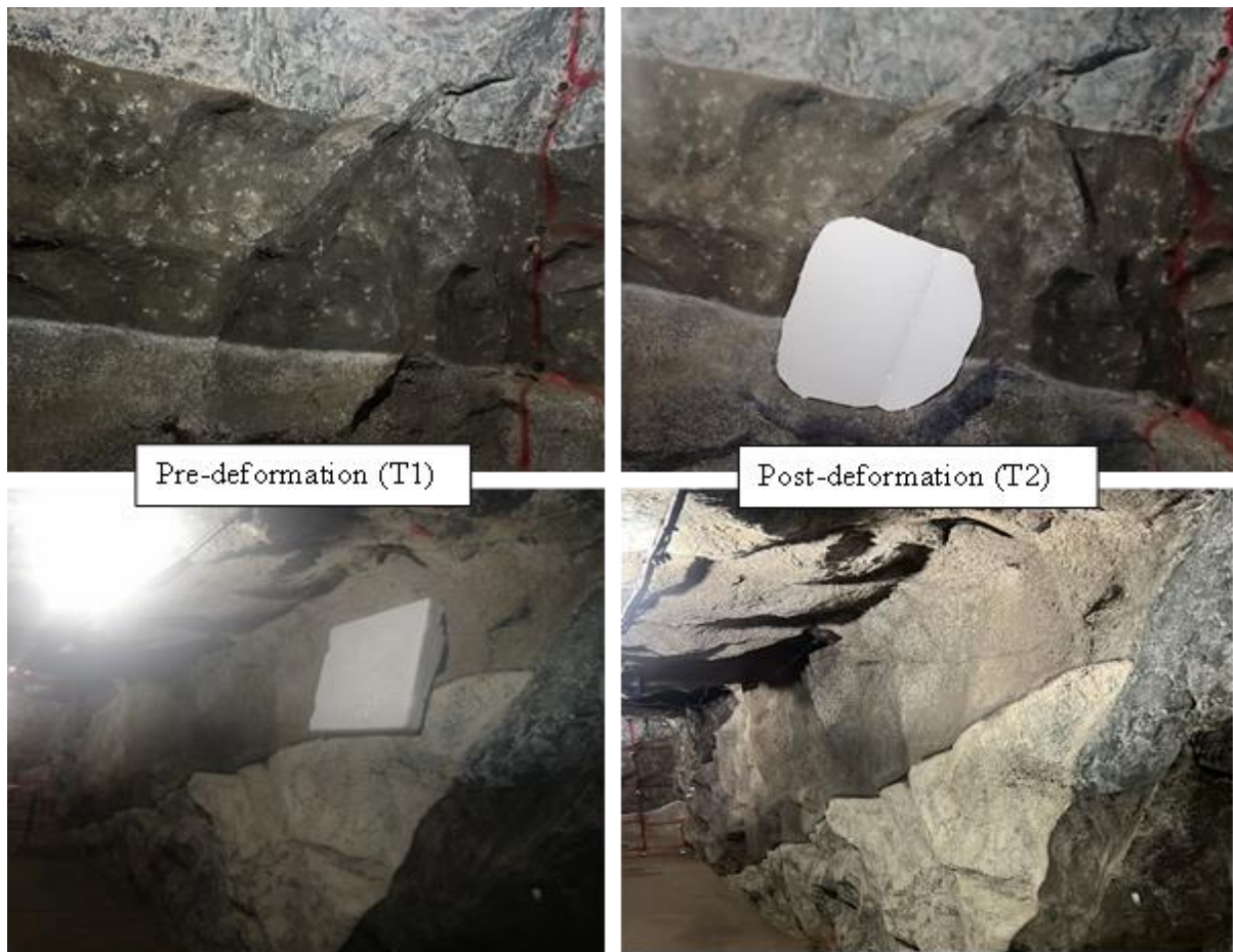
Figure 17: Underground tunnel displaying pre-and post-deformation simulation for rock burst scenario on the tunnel's rock surface
