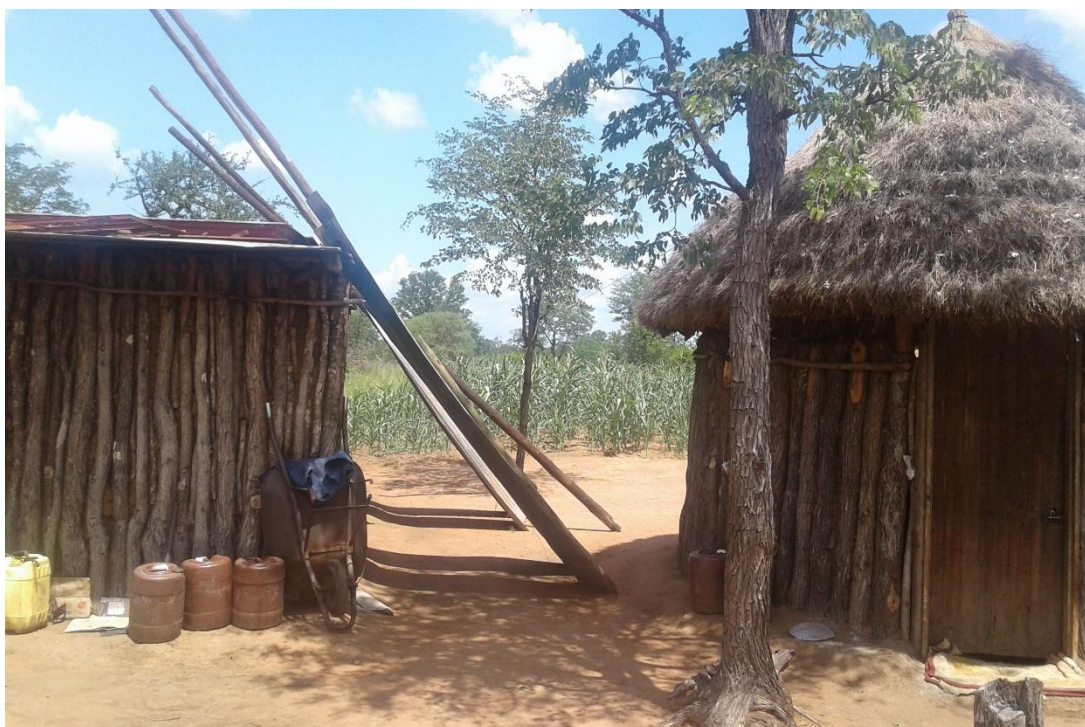
Picture 5.1 Houses constructed with poles and dagga in one-hectare plots (Source: Author)
