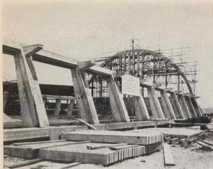
LEFT: The R.C. End frame with the inclined arch rib abutments. On the ground are the precast units which formed the panels of the lower retaining wall between the abutments. RIGHT: The "three-pinned" precast reinforced concrete arch ribs and tie beams in position. At left is the lean-to structure over the rail siding.
