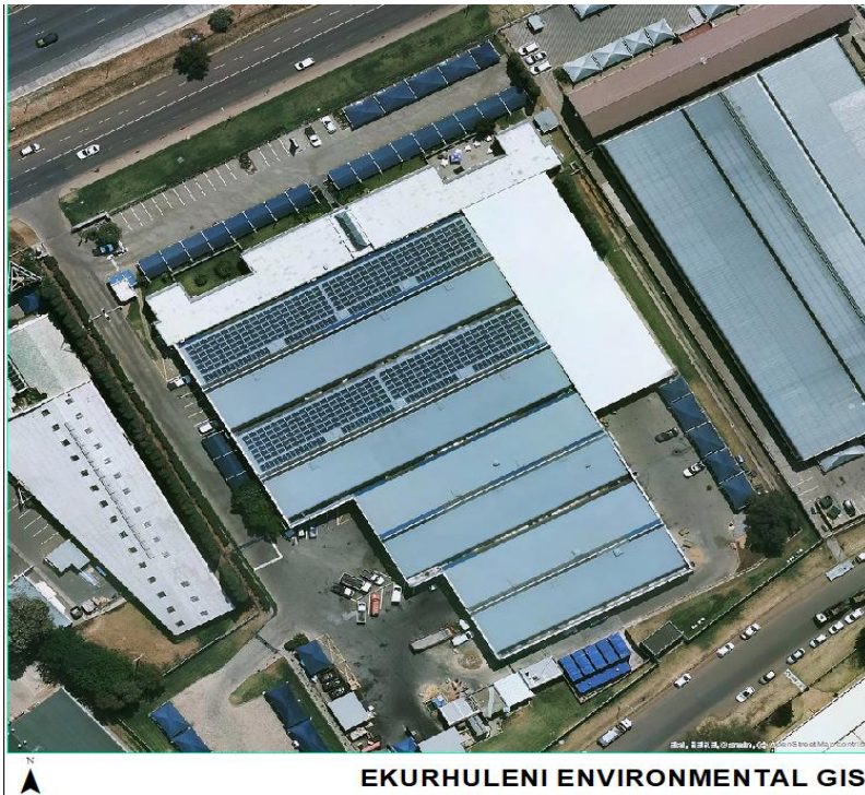
Figure 2: High-resolution image of an industrial neighbourhood, showing a solar installation.
