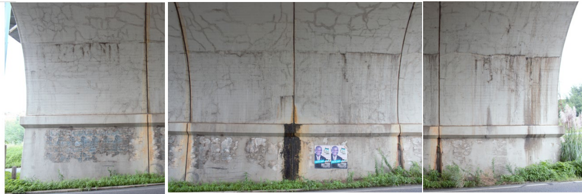
Figure 11: Pier 1 – Interior wall, facing eastwards
