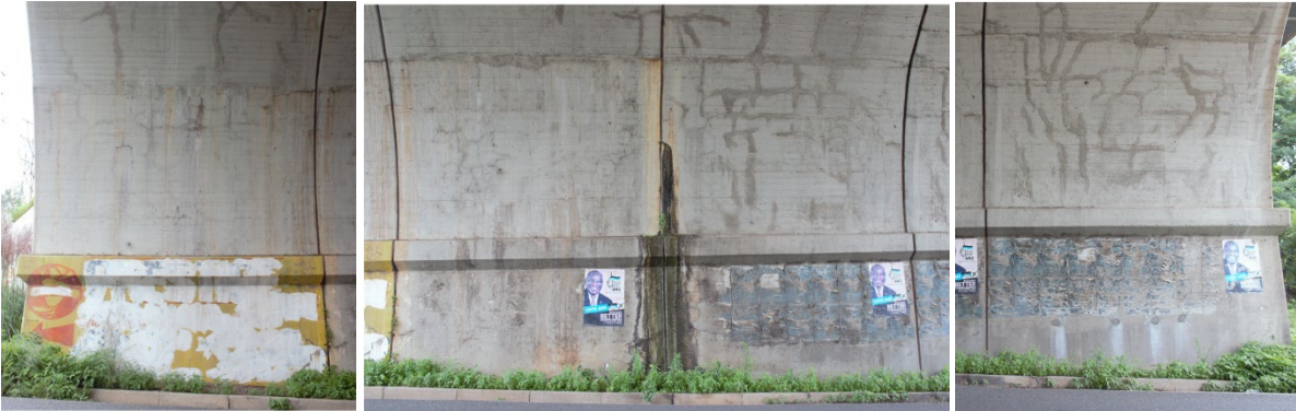
Figure 12: Pier 1 – Interior wall, facing westwards
