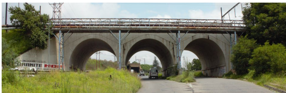
Figure 4-4: South-facing view of RC railway Bridge on Treu Road and Crown Mines Spur
