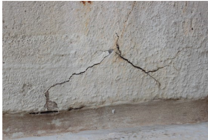
Figure 4-7: A greyish coating is seen on the exterior concrete surface of the entire RC railway bridge.
