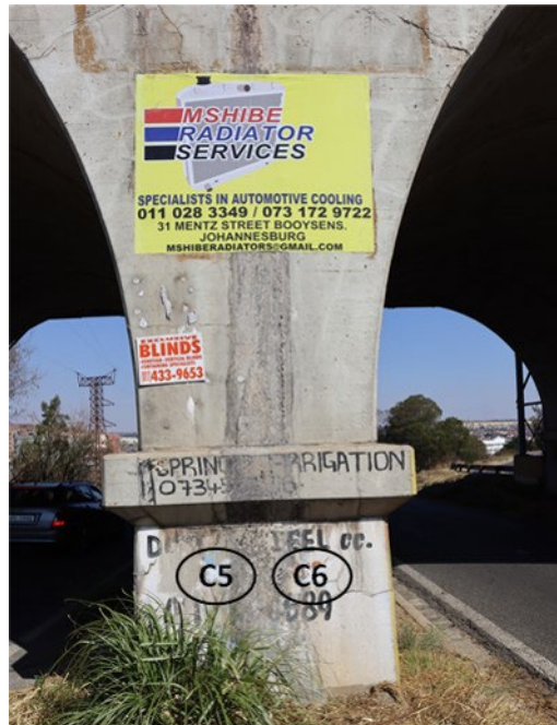
Figure 4-9: Location where cores C5 and C6 were extracted from Pier 1 – North-facing
