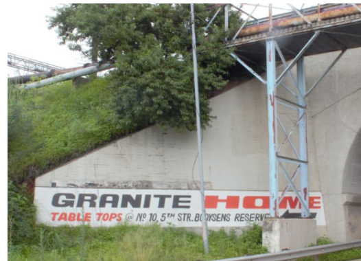
Figure 7: Abutment 2 – Southwards facing side
