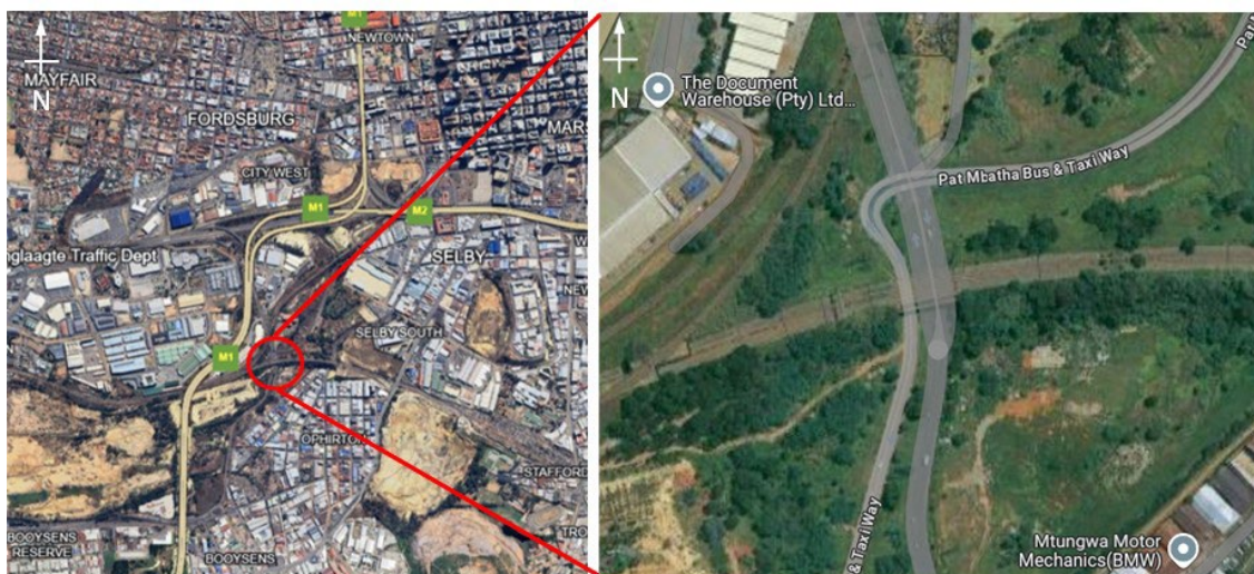
Figure 4-1: Geographical location of the RC railway bridge in Johannesburg (GPS co-ordinates 26°13'13.4"S 28°01'31.3"E)
