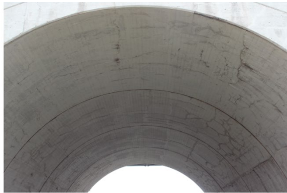
Figure 16: Arch 1 (View from North side looking Southwards)
