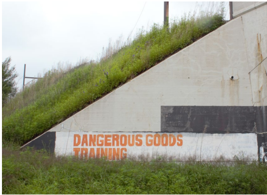
Figure 4: Abutment 1 – Northwards facing side
