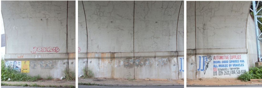
Figure 10: Abutment 1 – Interior wall
