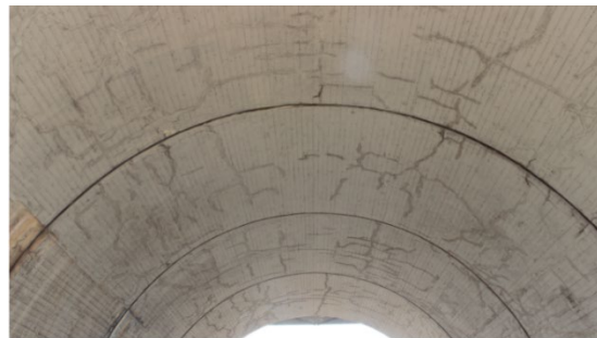
Figure 17: Arch 2 (View from the North side looking Southwards)
