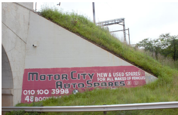
Figure 6: Abutment 2 – Northwards facing side
