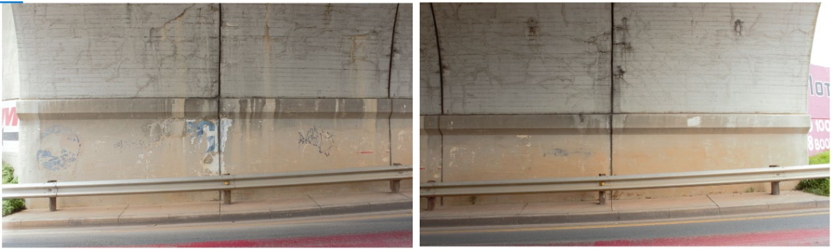
Figure 15: Abutment 2 – Interior wall
