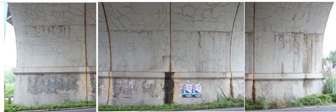
Figure 11: Pier 1 – Interior wall, facing eastwards
