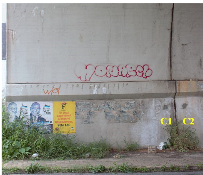
Figure 4-17: Location of core C1 in relation to location of C2 from Abutment 1- inner wall
