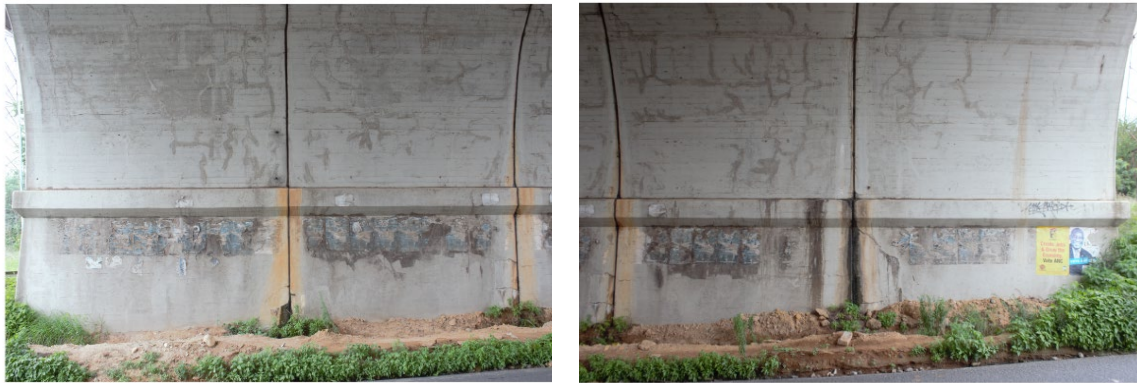
Figure 13: Pier 2 – Interior wall, facing eastwards
