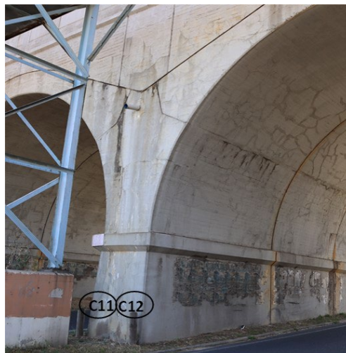
Figure 4-11: Location where cores C11 and C12 were extracted from Pier 1 – South-facing
