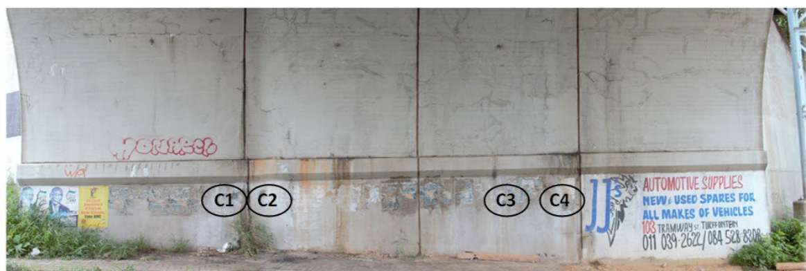
Figure 4-8: Location where cores C1, C2, C3 and C4 were extracted from Abutment 1- inner wall
