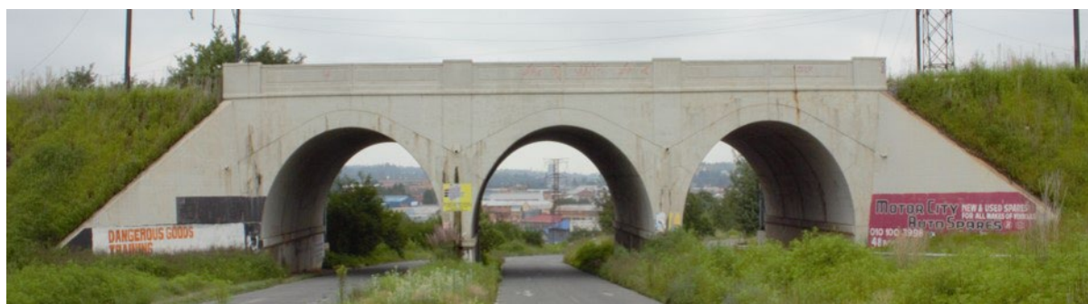
Figure 4-3: North-facing view of RC railway Bridge on Treu Road and Crown Mines Spur
