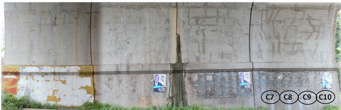
Figure 4-10: Location where cores C7, C8, C9 and C10 were extracted from Pier 1 – Interior wall, facing eastwards
