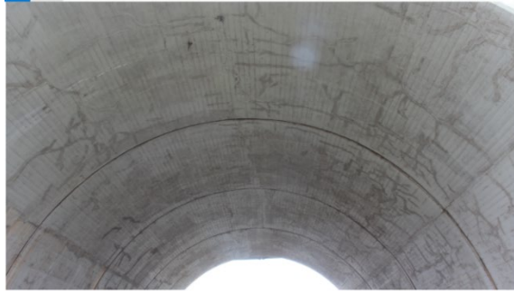
Figure 18: Arch 3 (View from the North side looking Southwards)
