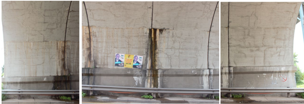
Figure 14: Pier 2 – Interior wall, facing westwards
