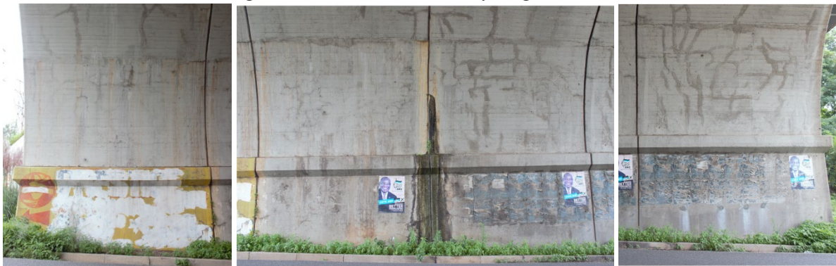
Figure 12: Pier 1 – Interior wall, facing westwards
