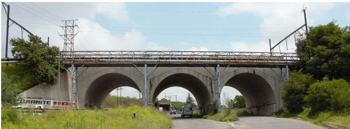
Figure 2: South-facing view of RC railway bridge located on True Road and in the Crown Mines Spur
