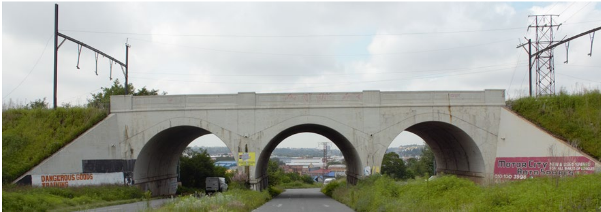
Figure 1: North-facing view of Railway bridge located on True Road and in the Crown Mines Spur
