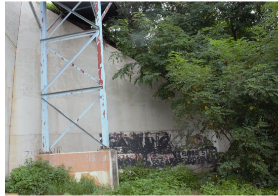
Figure 5: Abutment 1 – Southwards facing side
