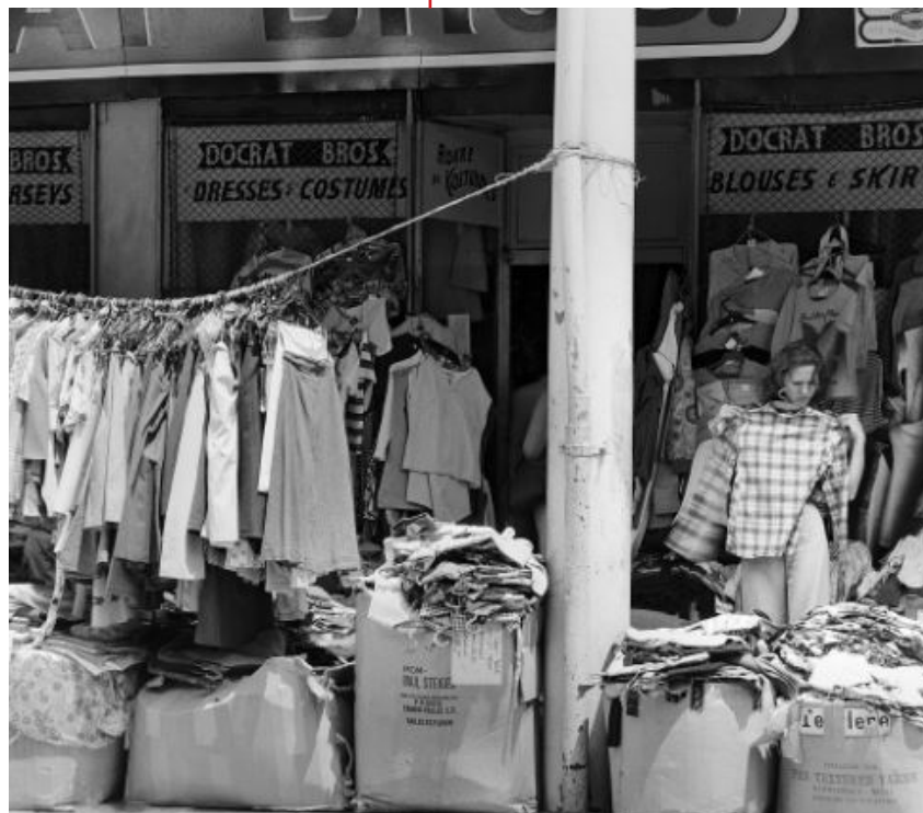
Fig 45 - Clothing shop on 14th street before the destruction under Group Areas Act in 1976 (Goldblatt, 1976)
