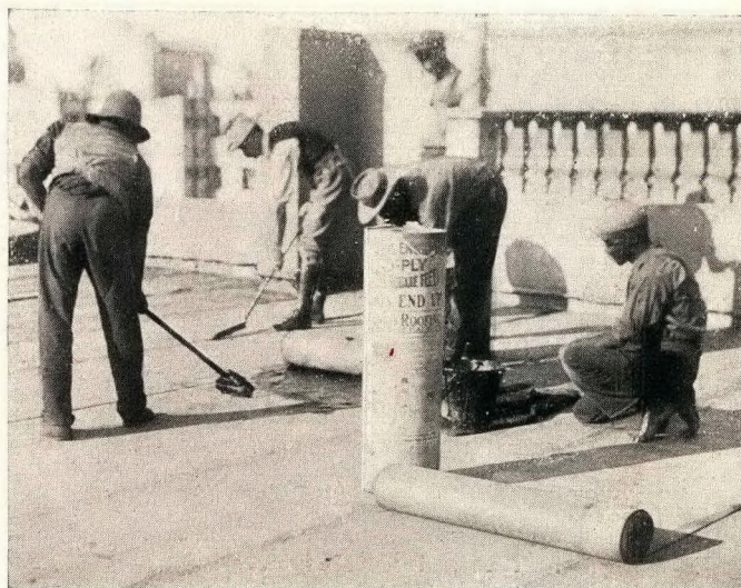
Showing Asphalte Work—Laying a new flat Roof to RAND CLUB, Johannesburg
