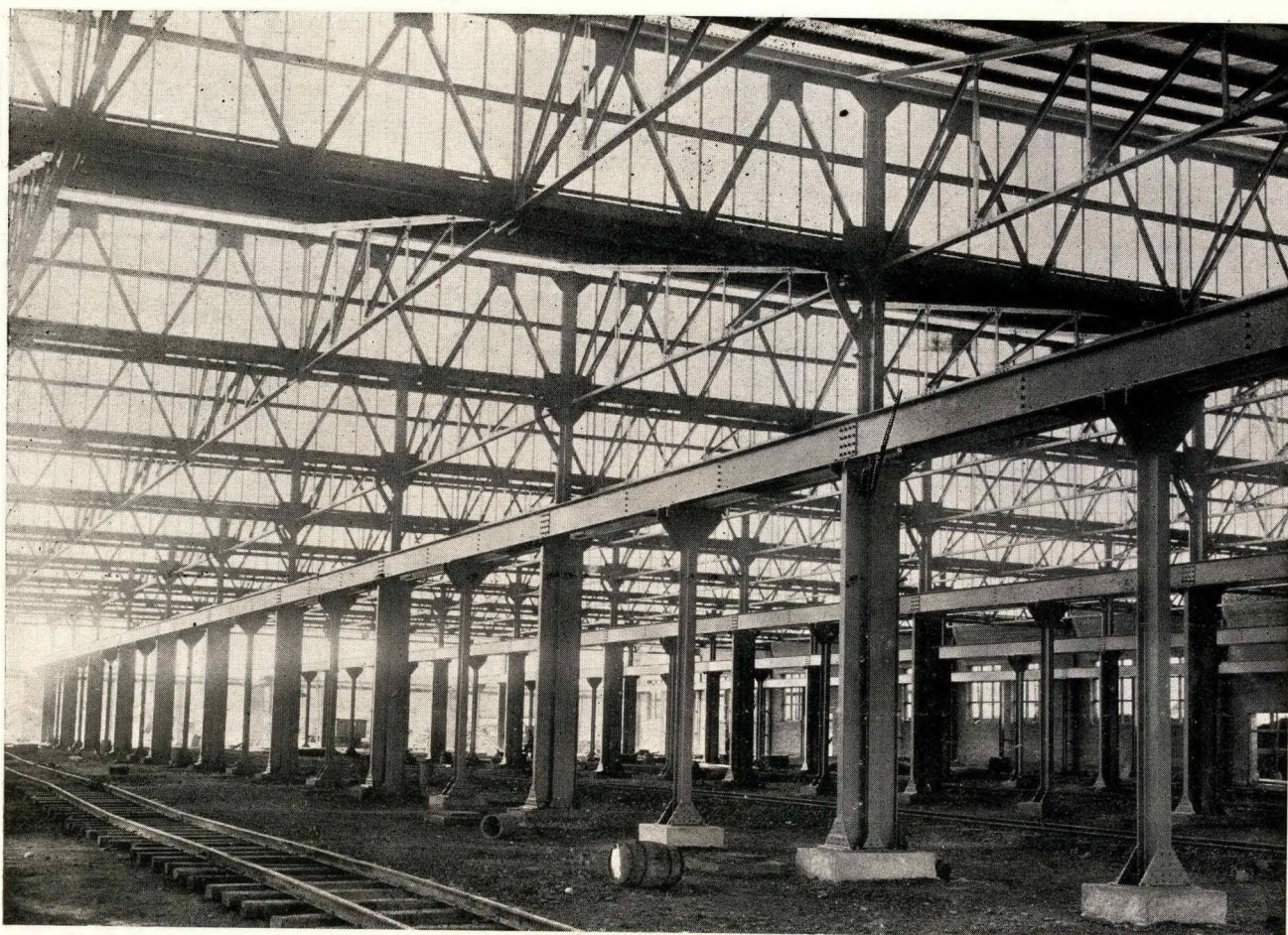
Internal View New Waggon Shops, S.A.R., Maritzburg. Total Weight of Structural Steelwork, nearly 1,000 tons. Supplied and erected by us complete.
