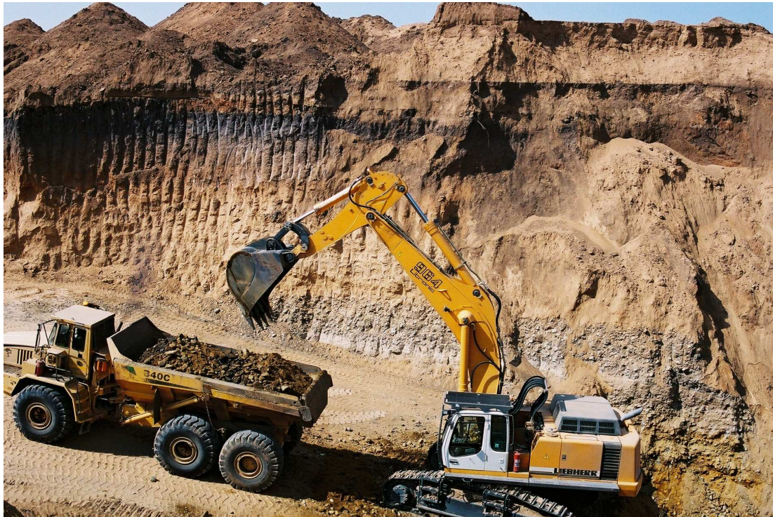
(a) Sydney-on-Vaal Pit 1. Dating sample collected from the base of the lower coarse alluvium.
