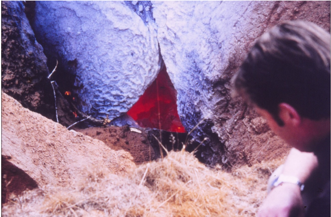
Figure 3.10 Partial collapse of a burning bord and pillar intersection (Photograph taken by Phillips)
