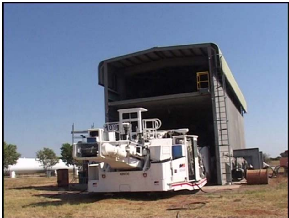
Figure 6.26 CM about to enter 20m tunnel (Courtesy of Mr Isaac Mthombeni)
