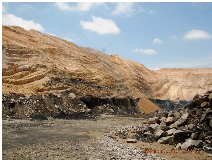
Figure 3.18 A highwall clad with soft, sandy material (Source: Phillips, Chabedi and Uludag, 2010)
