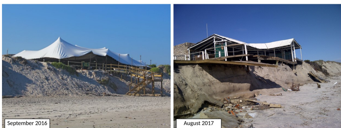
Figure 1.1: Comparison of before and after the June 2017 storm, which damaged the dune cordon and infrastructure along the southern section of Sixteen-Mile Beach. (Sources: left photograph from Dance Floor Hire ( www.dancefloorhire.co.za/project/strandkombuis-wedding/strandkombuis-wedding-2/ ), right photograph by Duncan Miller, used with permission).
