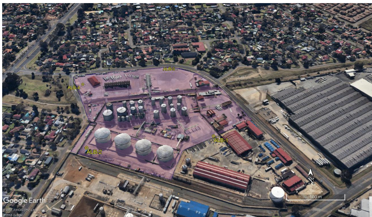
Figure 4.4: The Alberton depot (highlighted in pink) and labels indicating the sampling points. The Witbank site was surrounded by factories such as Samancor, Scew metals groups, Glencore alloys, suburb of Ferrobank and coal fields around the site (Figure 4.5).
