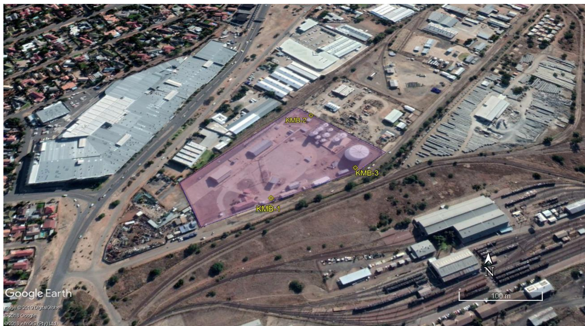
Figure 4.7: Kimberley depot with surrounding facilities and labels indicating the sampling points.
