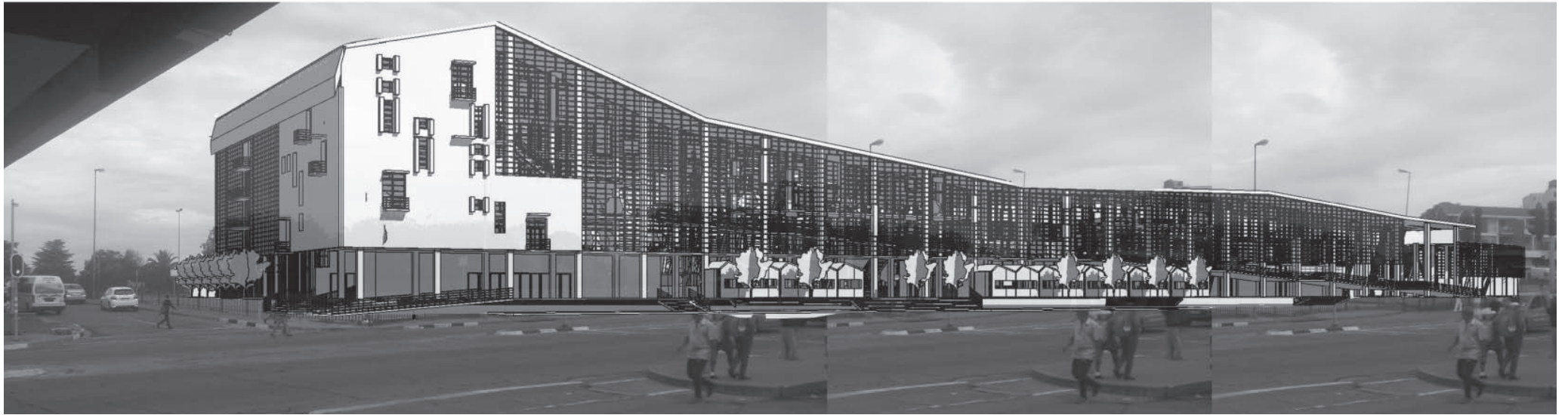
View of the Immigrant Integration Center from across Bram Fischer Drive
