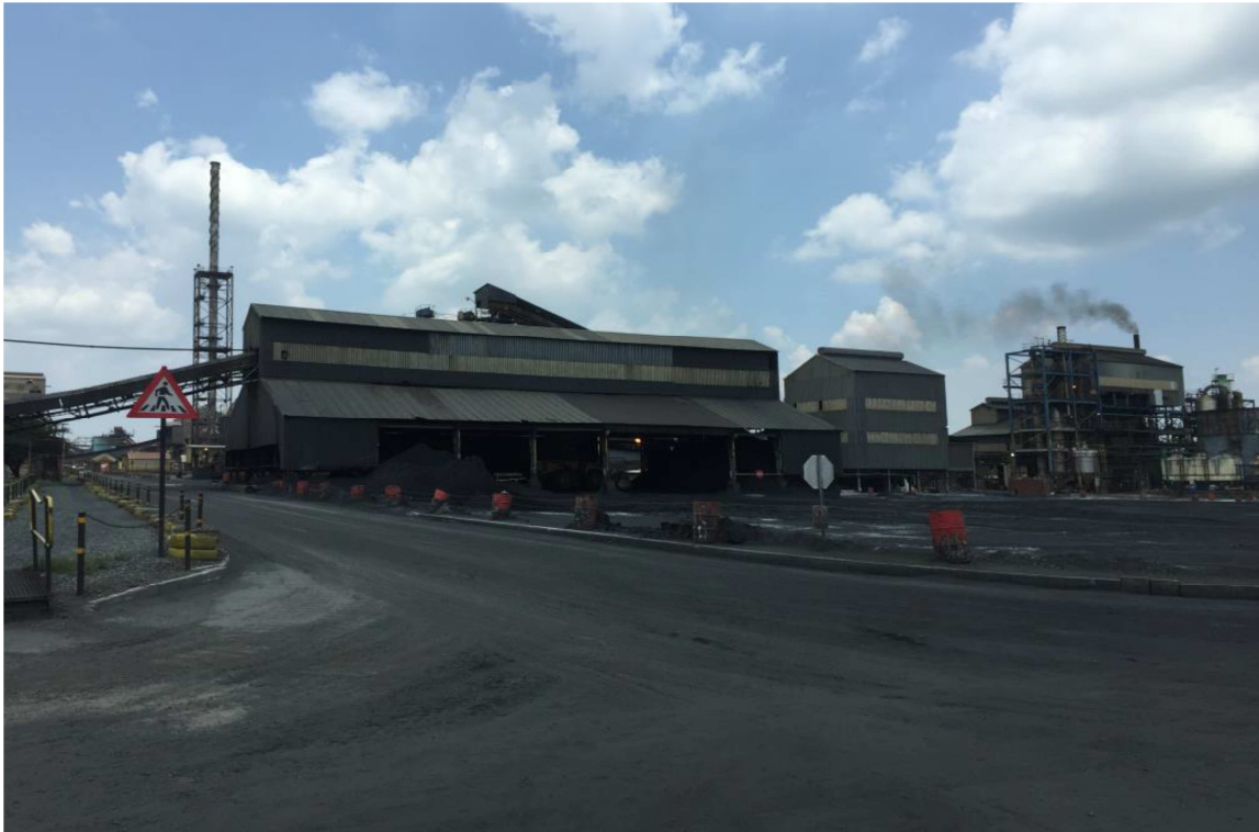
Figure 13: Vametco processing plant (Source: Bushveld website)
