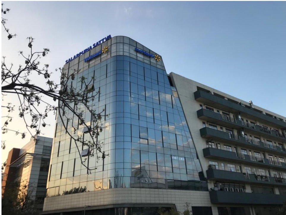
Figure 5.5 Walmart head office on outer ring road built by Salarpuria Sattva
