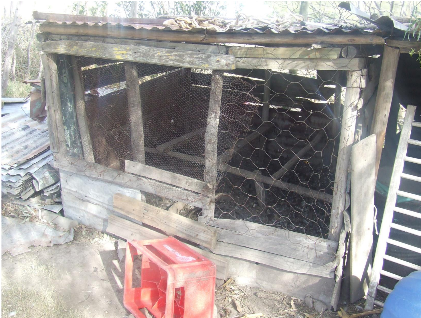
Figure 5.3: An example of a village chicken housing structure in the villages of Musina Local Municipality, northern South Africa. Housing structures were constructed with corrugated iron sheets, wooden poles and wire mesh. Photo by Njongenhle M. B. Nyoni.
