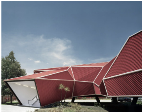
Figure 3.51: Nestle Chocolate Museum - the portal frame is placed inside the building envelope, aslo Sainsbury Centre and Great Glasshouse (Karmatrendz, 2009).
