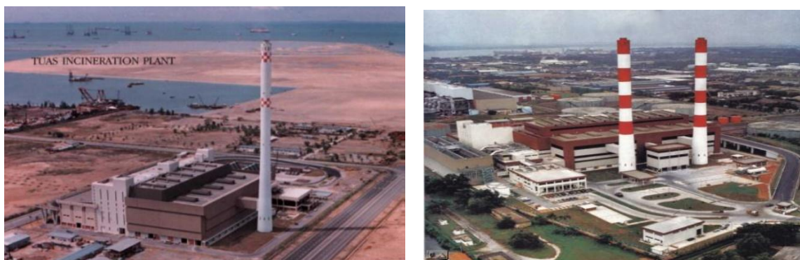
Figure 6: Tuas and Senoko Incineration Plants. Built in 1986 and 1992 respectively (Eng, 2012).
