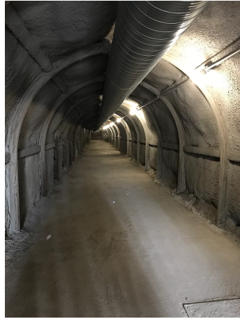
(a) The tunnel region of the WITS Mock Mine. The ventilation pipe can be seen on the ceiling.
