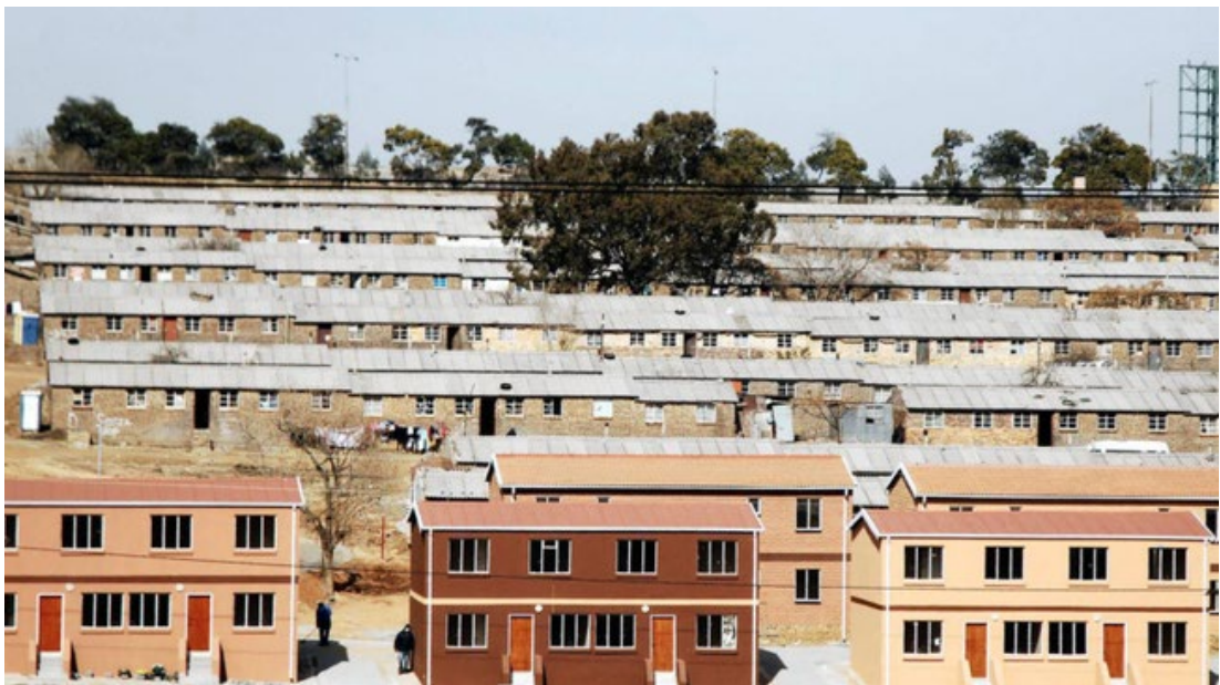
Figure 3: Diepkloof hostel and new high rising flats that stand contrast to the old dormitory style hostel buildings. Source: https://www.iol.co.za/news/hostels-must-fall-says-housing-minister-1855516 . [Accessed: 27 March 2021].
