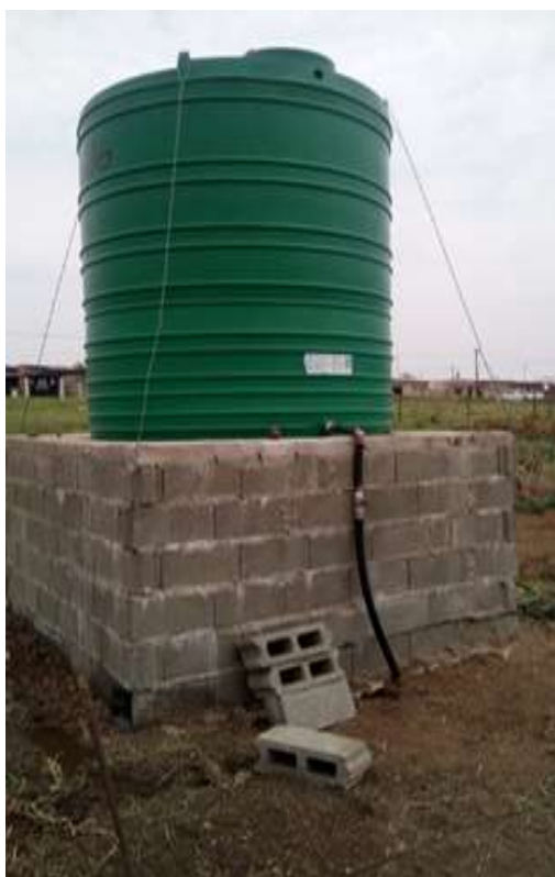
Figure 27: Image showing the new Jojo Tank
