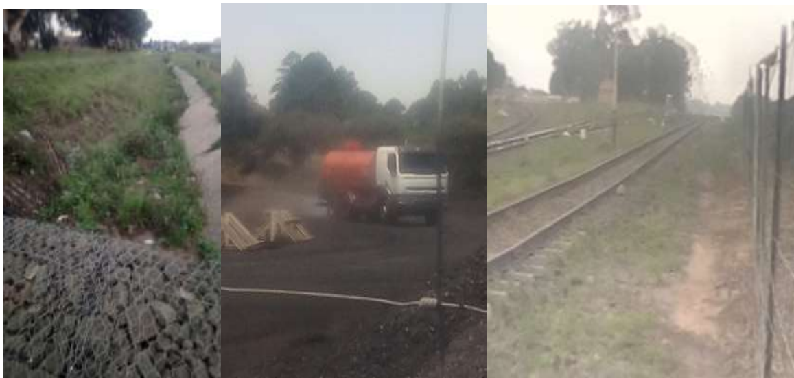
Figure 23 (i-iii): Images showing the small stream where the coal is washed into and the coal siding in Carolina
