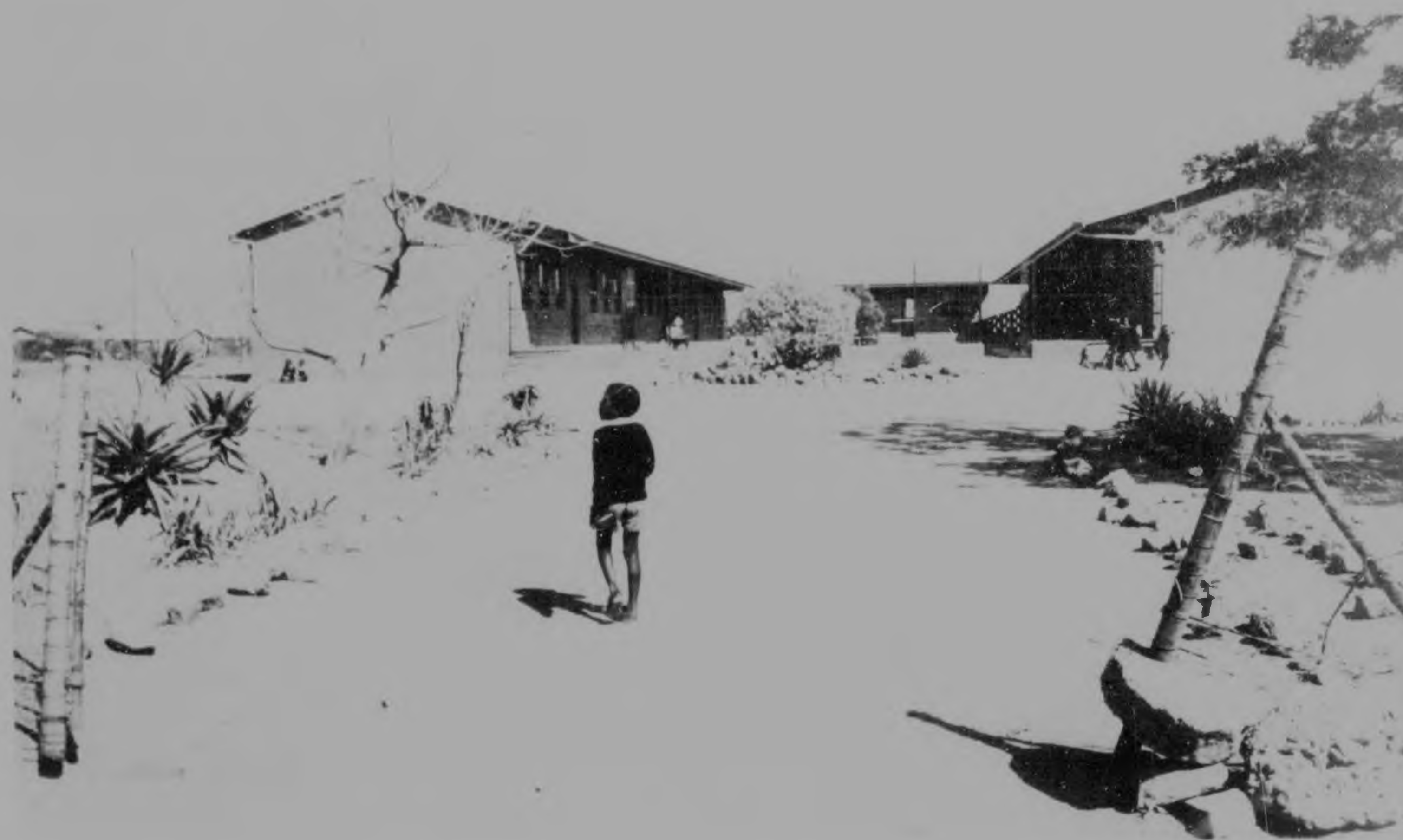
Mabopane school is a building situated in space and does not form part of the urban grain.
