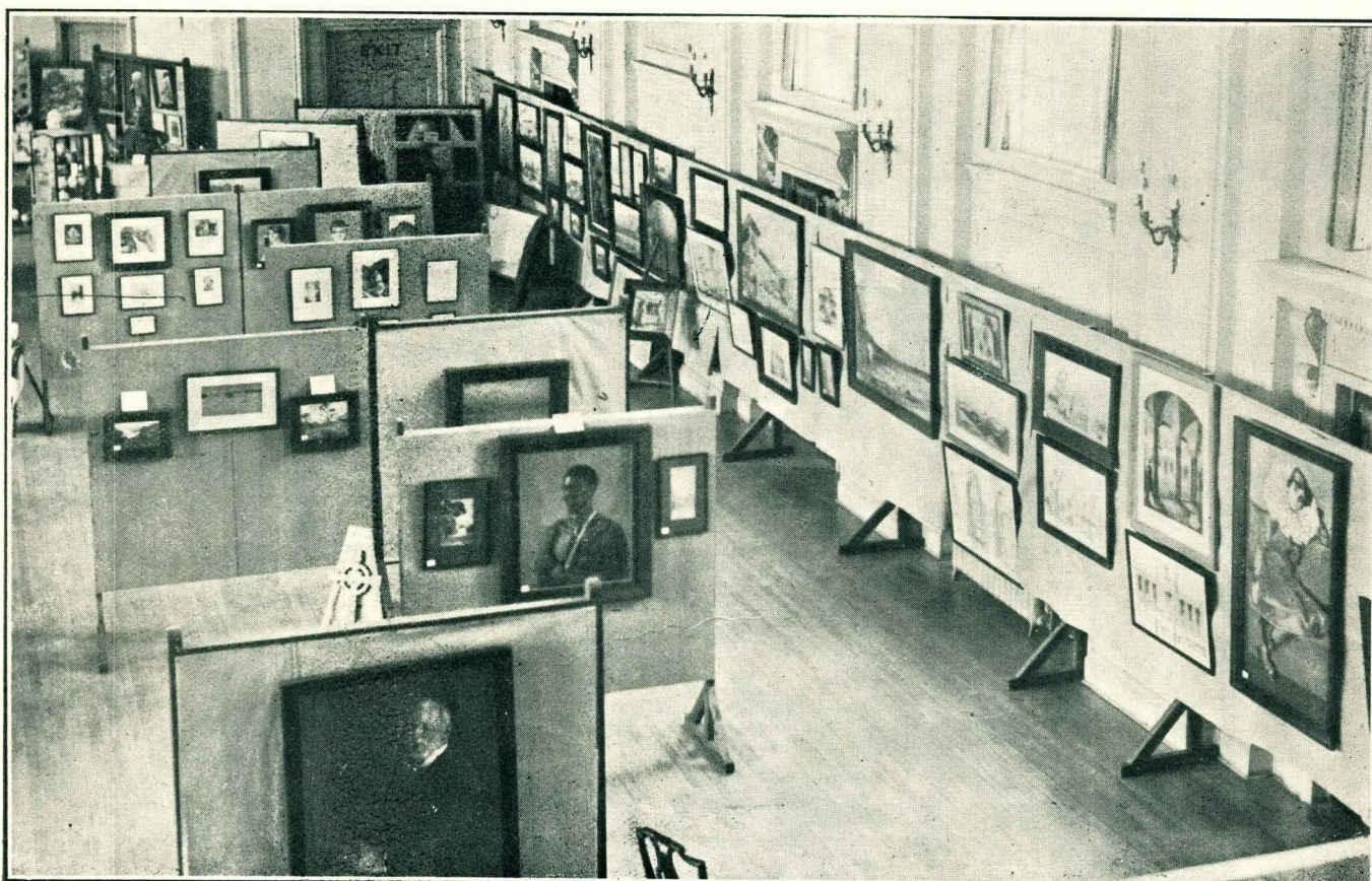
Two views of the first Exhibition held in the Selborne Hall, Johannesburg, under the auspices of the Association of Transvaal Architects.
