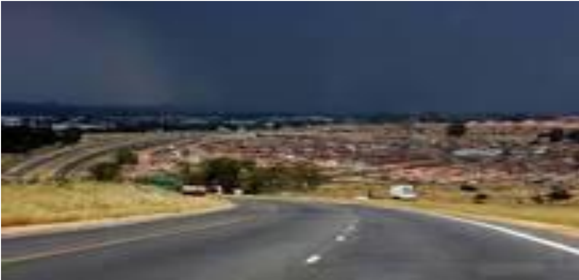
Figure 3: Various Infrastructure in Cosmo City
