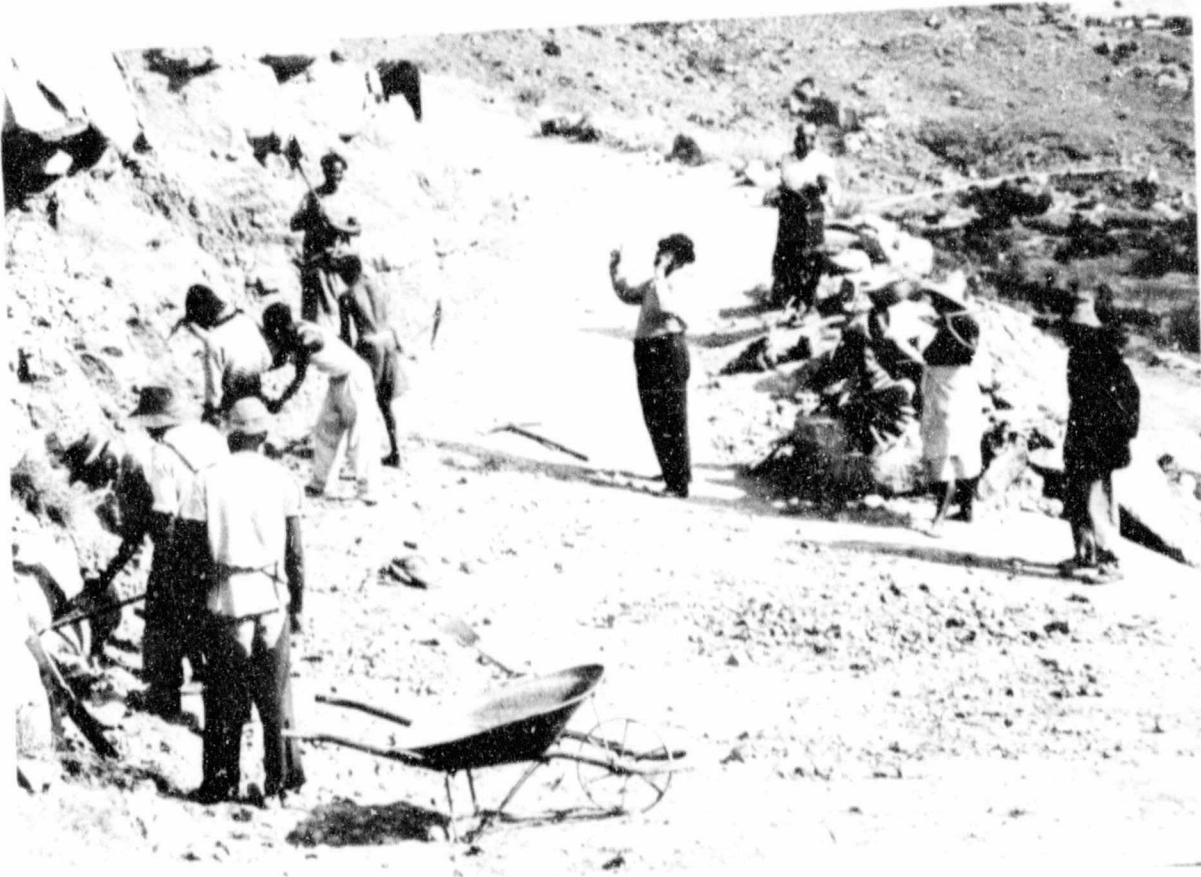
JOHRE CONDUCTING A VOLUNTARY ROAD IMPROVEMENT GANG ON THE APPROACH TO THE VALLEY.
