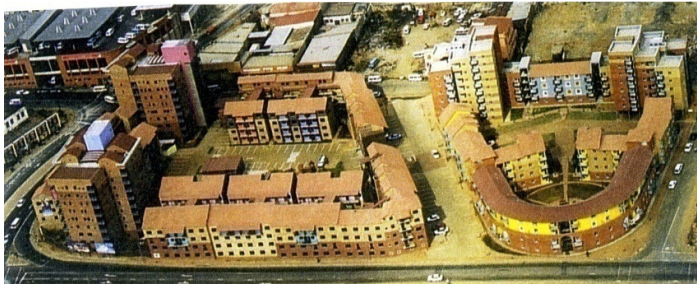
Aerial photograph 1a: Brickfields Precinct (on the left) and Legae Gardens (on the right - a yellow building) Source: JHC, 2005
