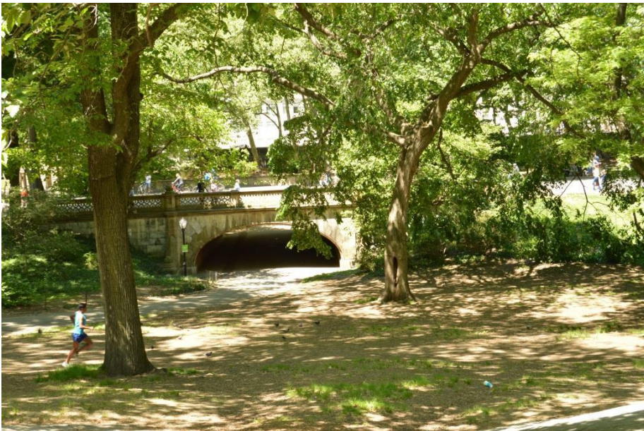
Image 54: Bridges and walkways adding to the environmental setting of Central Park (Shelton, 2015)
