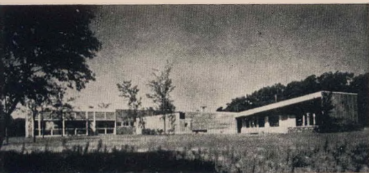
The living room wing is on the left, the guest house is on the right.
