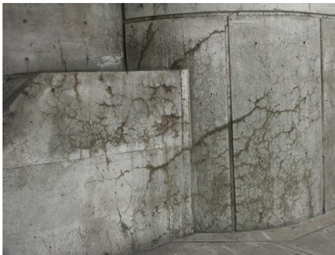
Figure 4: Sidewalk level of large concrete elements showing signs of serious ASR damage.
