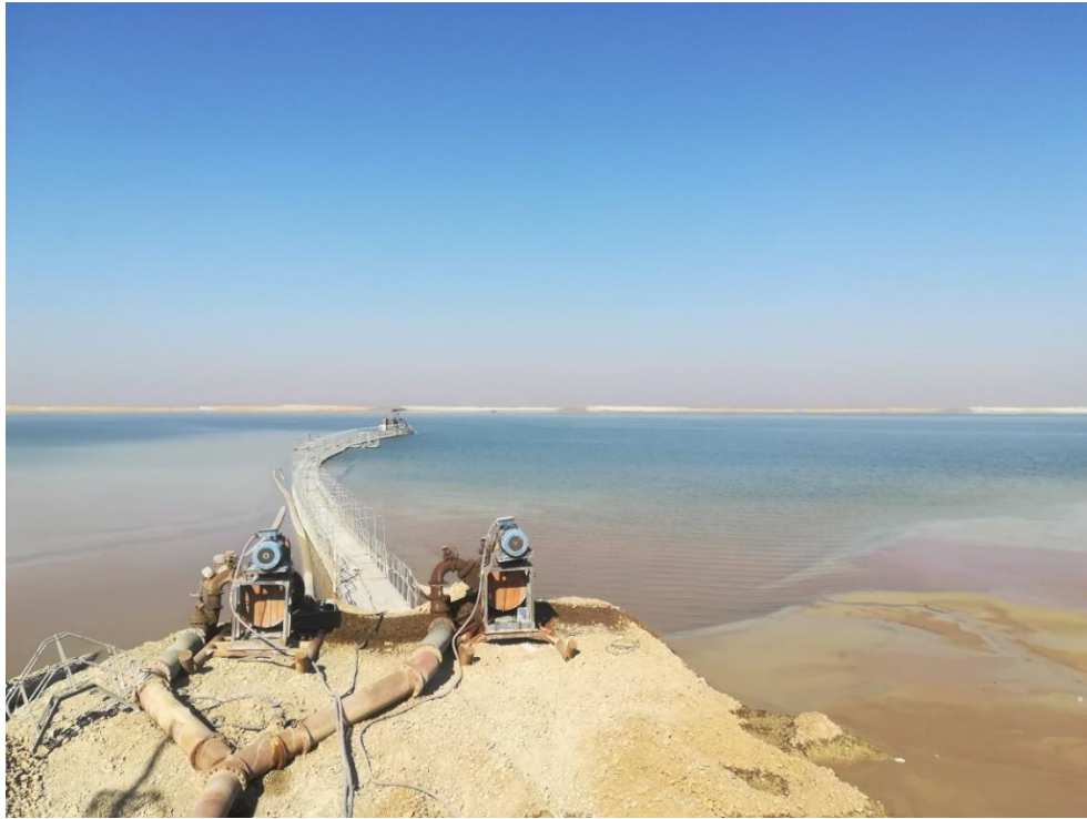
Figure 3.3. A photograph taken before the catwalk, at the top of Site B's tailings storage facility.
