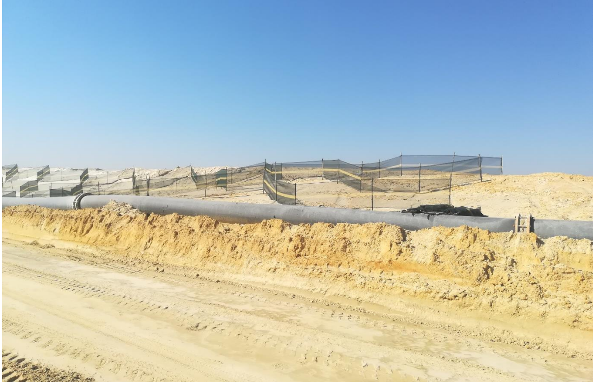
Figure 4.6. Netting used to prevent dust fallout as a result of wind.
