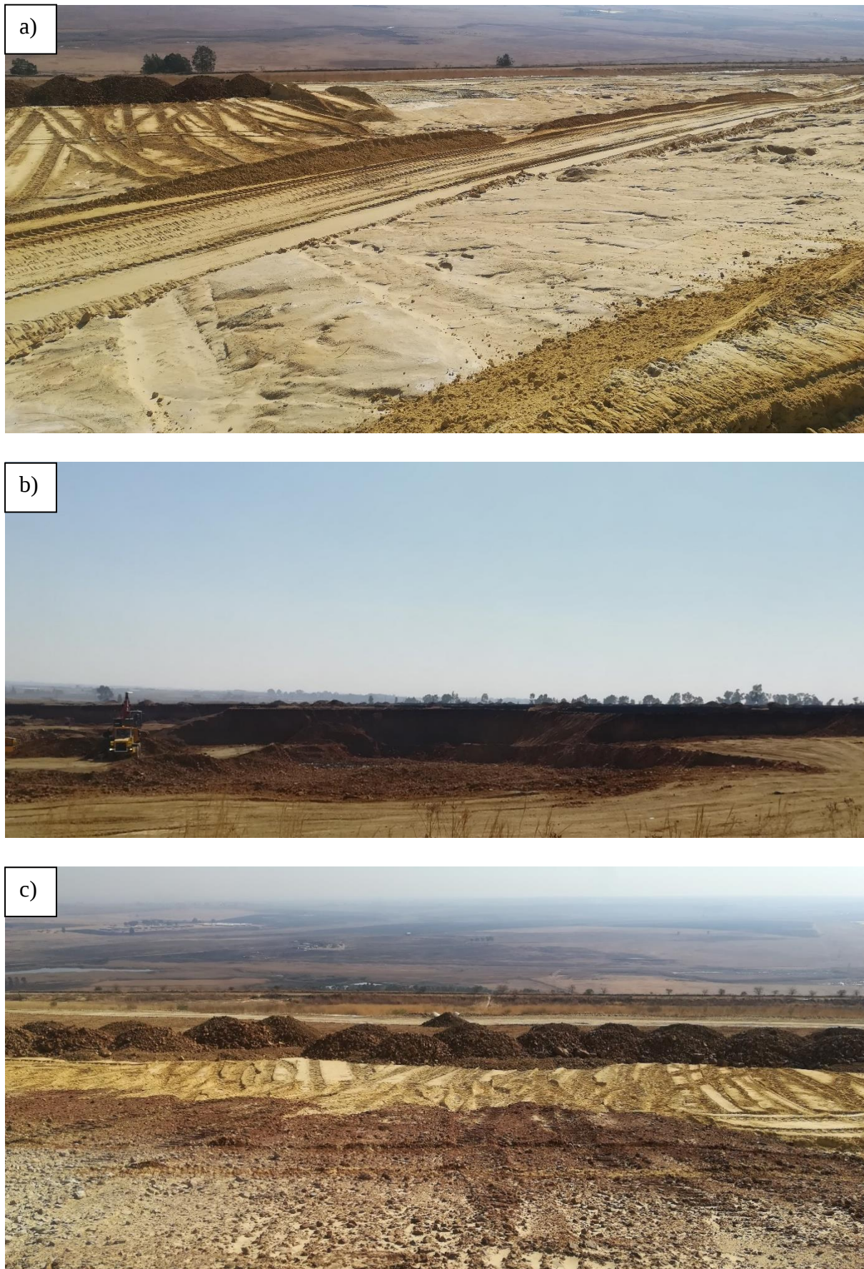
Figure 4.5. A photograph taken from the top of a slope being prepared for cladding.
