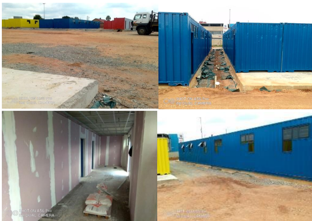
Figure 4. 7: Marlboro Container Housing Units as of 16 December 2020, all work on heavily reinforced slab. Source: Author's, 2020
