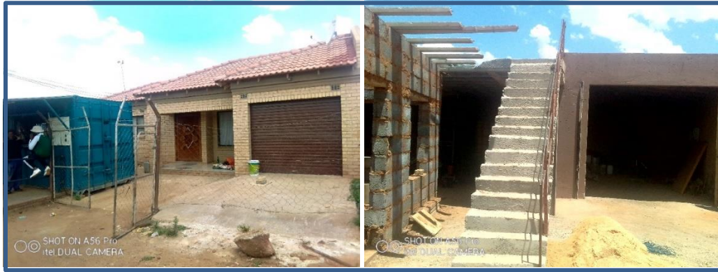
Figure 4.13: A newly constructed house in Slovo Park (left photo) and a double-storey residential building under construction (right photo): Source: Author, 2020
