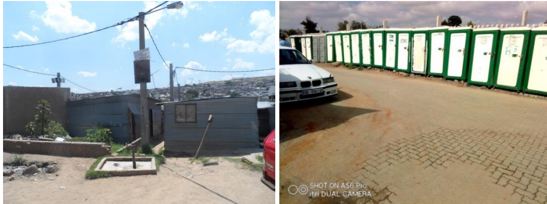
Figure 5.4: Communal water standpipe (left photo), lockable chemical toilets located on the far western end outside the built area along the main access road into Stjwetla (right photo). Source: Author, 2021
