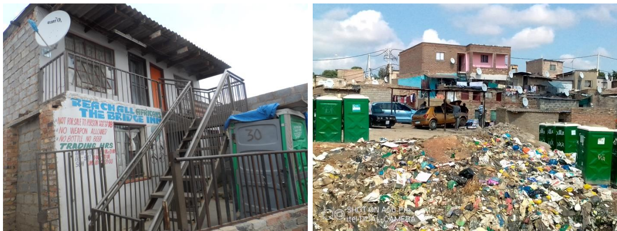
Figure 4.2 Storey brick-and-concrete residential and business structure (left photo) and another storey residential (right photo). Source: Author, 2020
