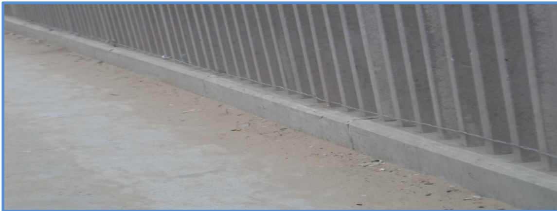
Figure 5.6: A typical illegal connection showing a live electric cable across the footbridge from the Alexandra East Bank developments to Stjwetla on the west bank: Source: Author, 2019
