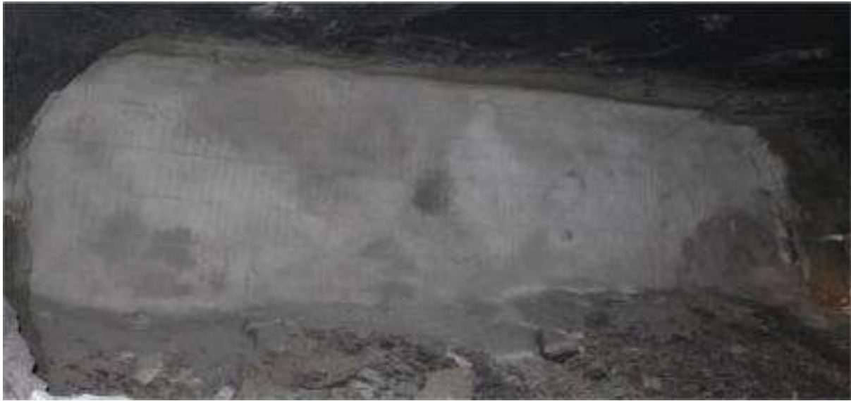
Figure 4.3: Example of a shotcreted pillar holing seal
