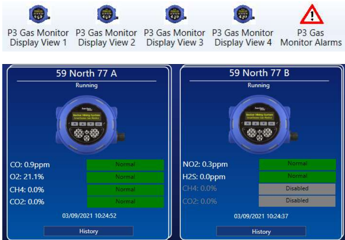
Figure 5.5: Real time gas monitoring at the mine
