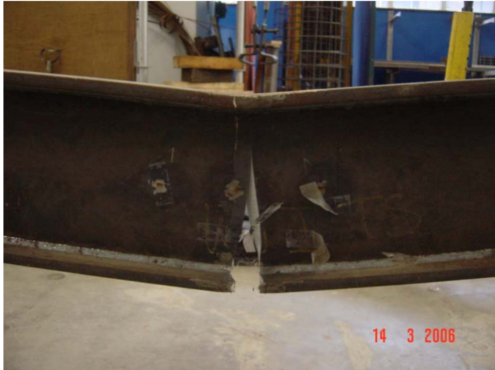
Figure 4.18b – Specimen at failure
